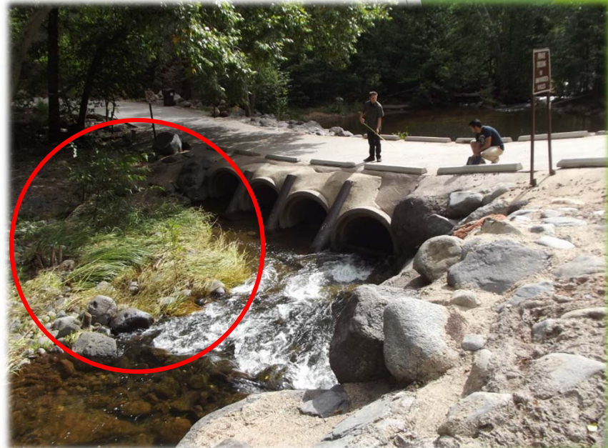
The soil deposit deflects the water to flow through the two culverts located closest to 89A
